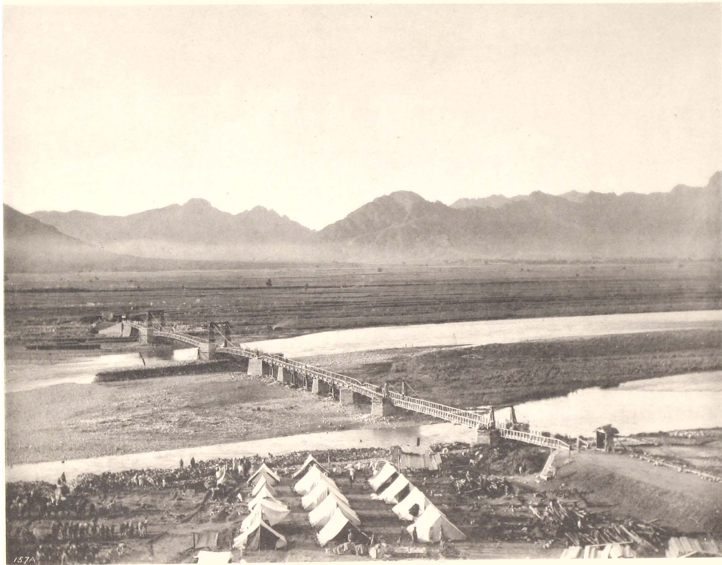
THE BRIDGE OVER THE SWAT RIVER,
