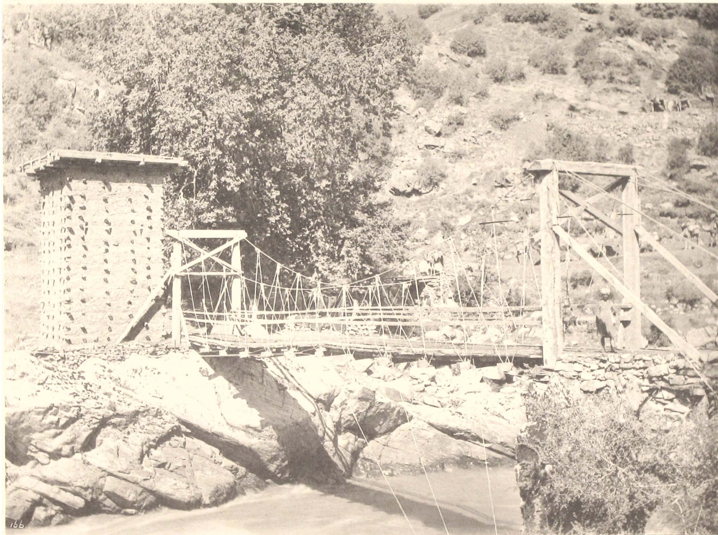
SUSPENSION BRIDGE AND BLOCK HOUSE OVER PANJKORA RIVER,
