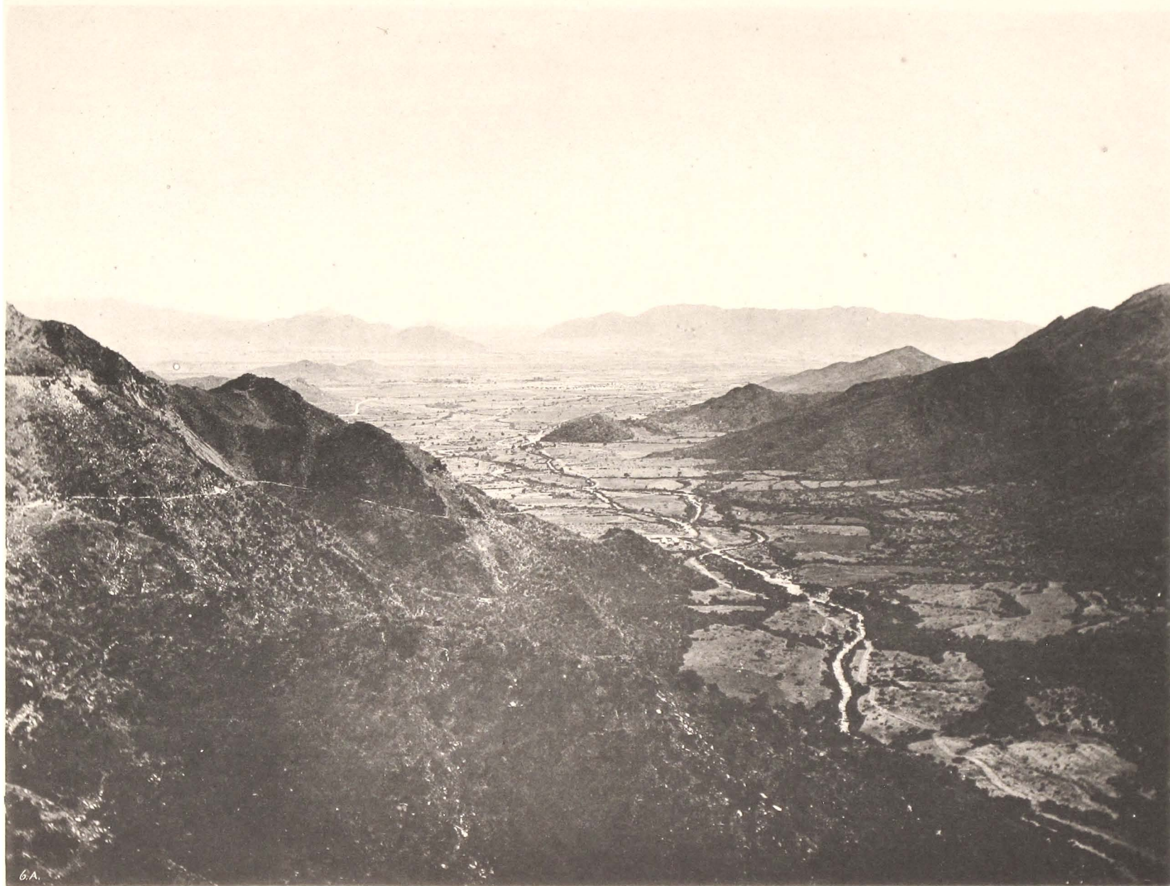
6A. BUDDIST ROAD, MALAKAND PASS, LOOKING SOUTH.
