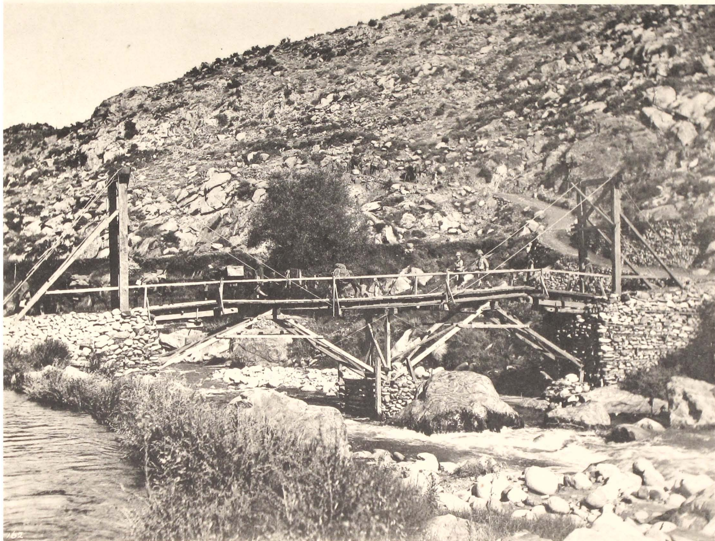
SUSPENSION BRIDGE, BETWEEN WARAI AND DARORA, IN PANJKORA RIVER.
